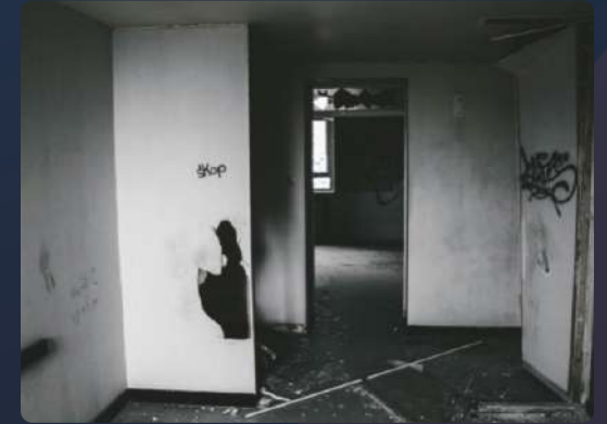
Interior of a dilapidated apartment with the front door in NYC
